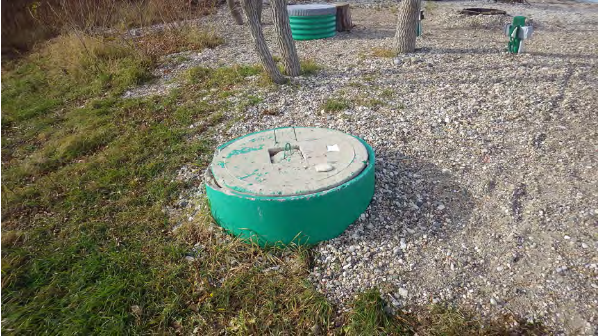
Figure 13: Underground tank access in the cleared area
