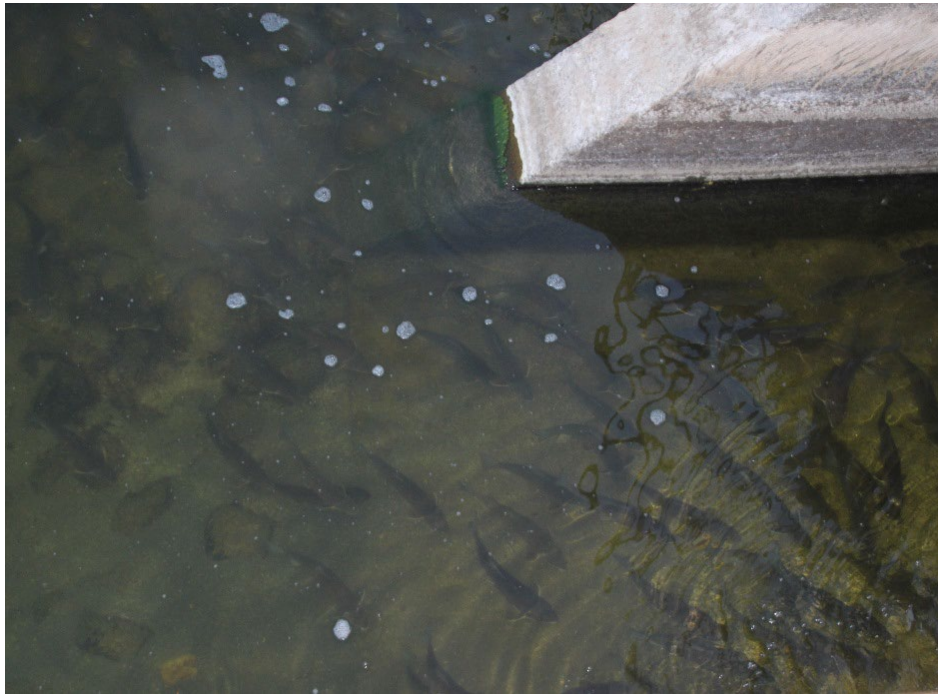
Photograph I-11 Fish congregating downstream of the existing outlet structure (May 19, 2016).
