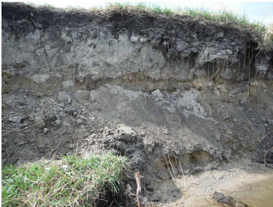
Photograph I-12 Erosion along the Qu'Appelle River (May 19, 2016).
