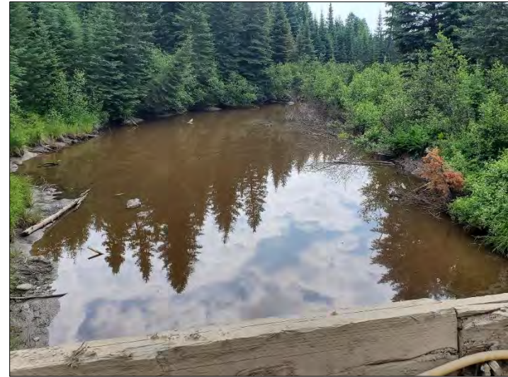
Downstream overview of Dixie Creek from the bridge in spring (June 2023)
