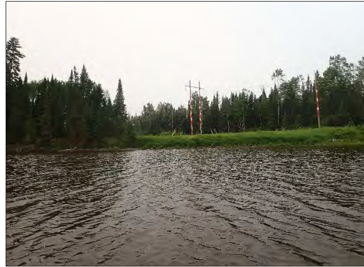
Overview of powerline crossing, facing north (June 2023)
