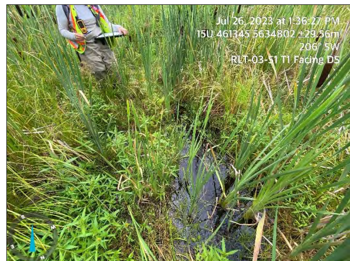
Narrow channel with minor scour and alluvial deposition (July 2023)
