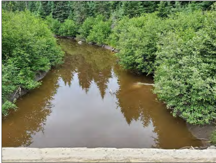
Upstream overview of Dixie Creek from the bridge in spring (June 2023)
