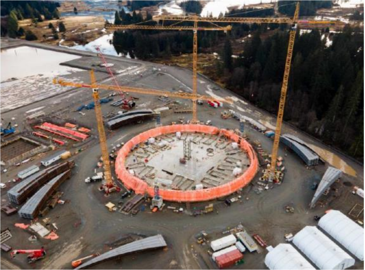
PHOTO 6: COMPLETED LNG STORAGE TANK CONCRETE GROUND SLAB (DECEMBER 2020)
