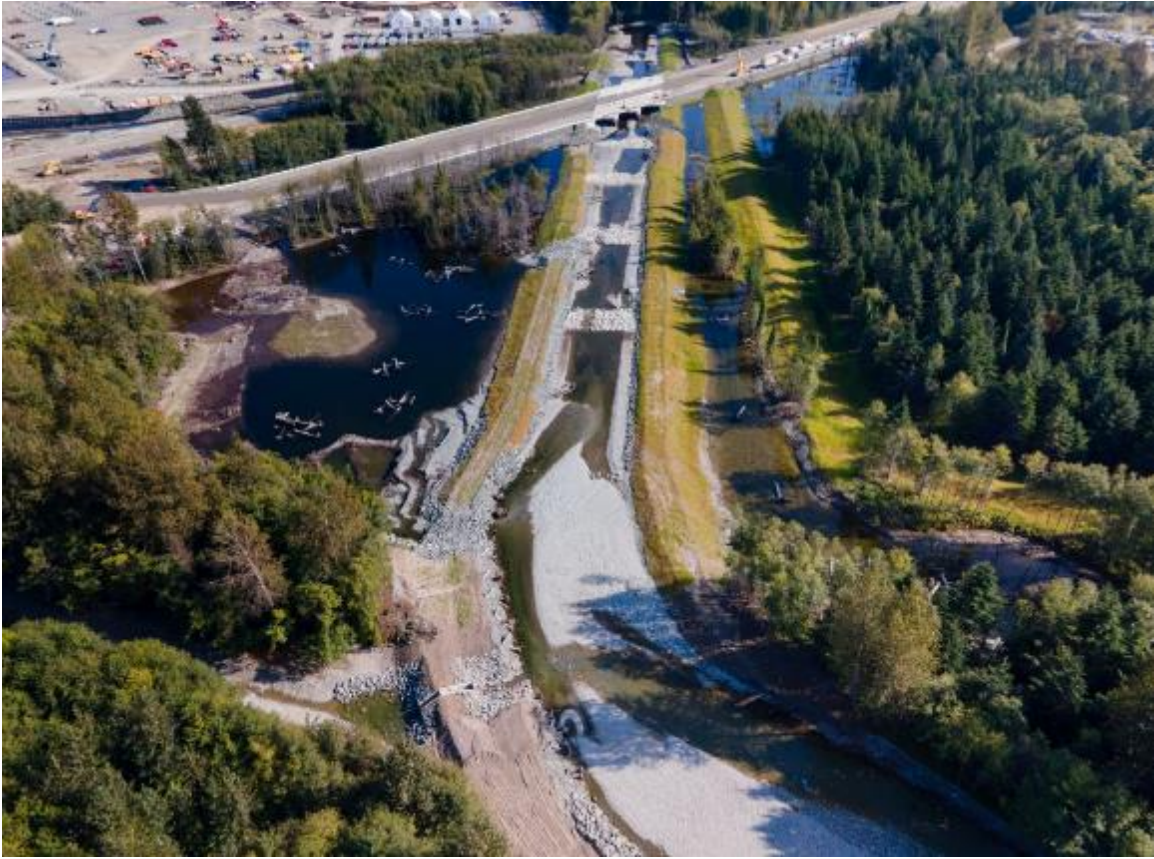
PHOTO 9 – ANDERSON CREEK RE-ALIGNMENT (SEPTEMBER 2020)
