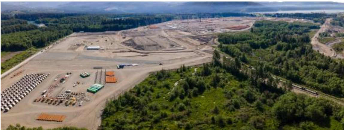
PHOTO 1: SITE PREPARATION ACTIVITIES (JUNE 2020)
