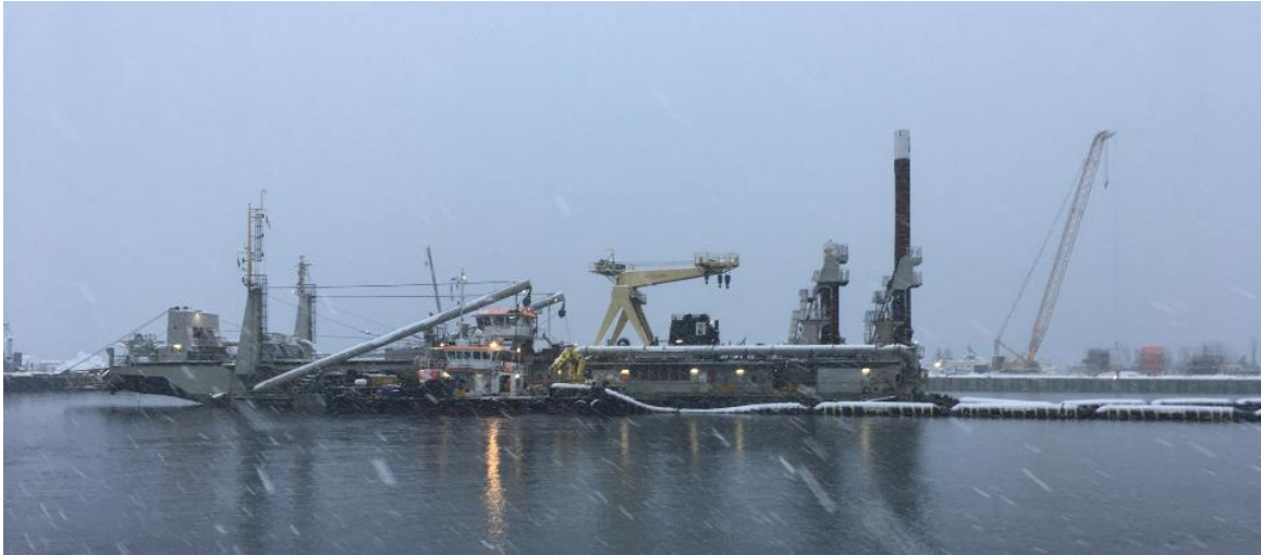
PHOTO 3: CUTTER SUCTION DREDGE (CSD) VESSEL (WINTER 2020/21) DREDGE VESSEL
