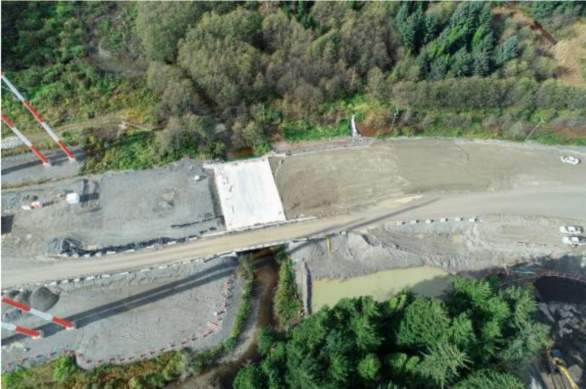
PHOTO 2: MOORE CREEK BRIDGE (OCTOBER 2020)
