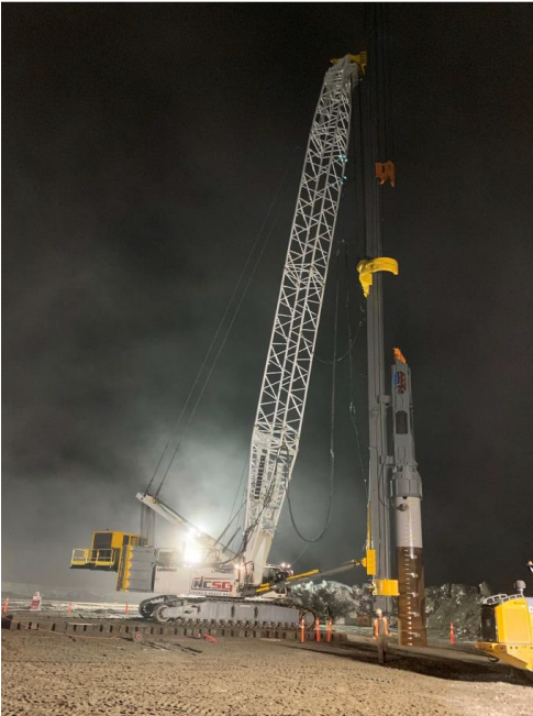
PHOTO 5: LNG FACILITY PILING (FEBRUARY 2020)
