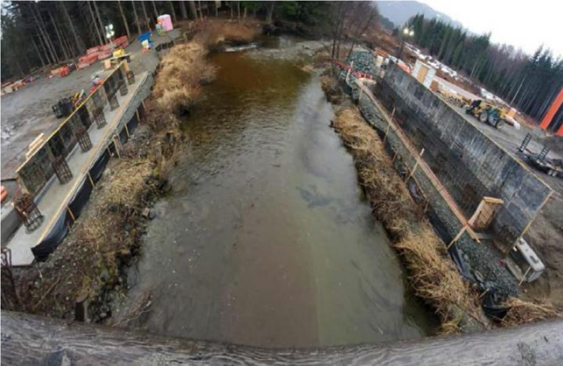
PHOTO 2: MOORE CREEK BRIDGE NOTH ABUTMENT FORMWORK INSTALLATIONS (MARCH 2020)
