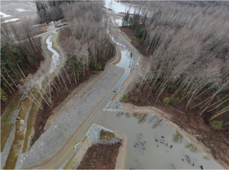
PHOTO 10 – CONSTRUCTION OF THE KRSC (KITIMAT RIVER IN TOP OF PHOTO) (NOVEMBER 2019)
