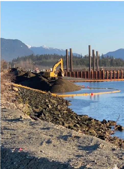
PHOTO 4: BACKFILLING THE WEST MOF; PILES AT NORTH MOF (MARCH 2020)
